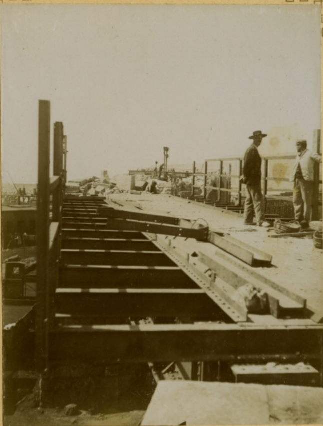
ALQUIFE PIER BRIDGE OVER BEIRES SIDING
