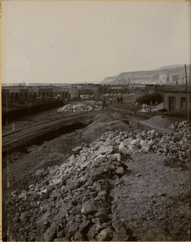
ALQUIFE PIER WORKS OCT 1902
