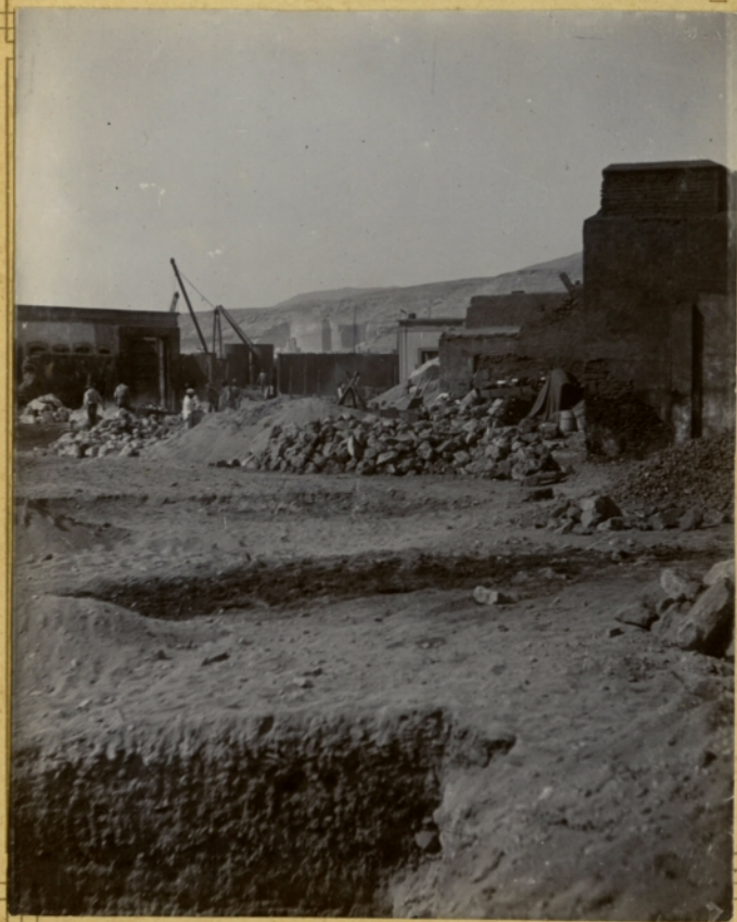
ALQUIFE PIER WORKS OCT 1902
