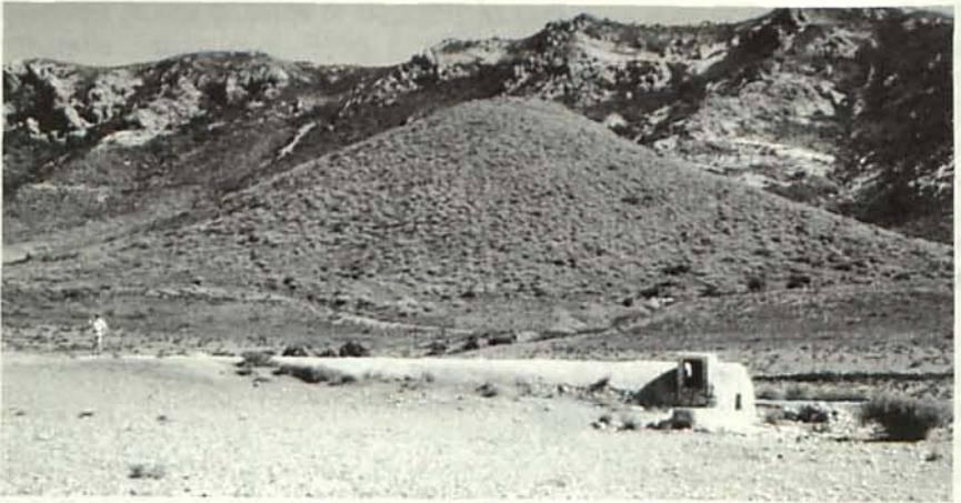
Figure 2. Position of a large aljibe ( 314 \text{ m}^3 ) with a catchment on a steep hillslope in the Sierra de Gata. Note the runoff conduits at the base of the hill leading runoff to the aljibe and the sediment cleared from the aljibe.
