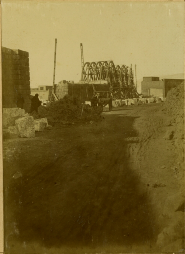
ALQUIFE PIER WORKS
