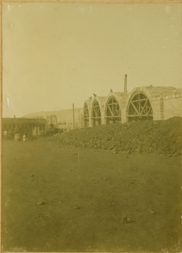
ALQUIFE 28/1/903 PIER WORKS
